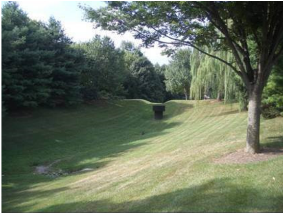
Detention (dry) basin
