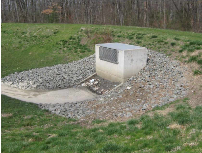
Riser in detention basin
