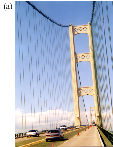
Cables of Mackinaw bridge
